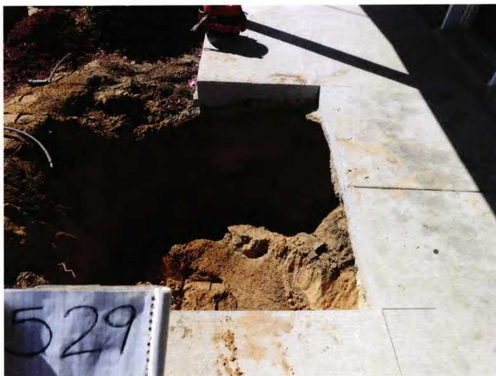
Picture 2: UST 529LaurelBB excavation.
